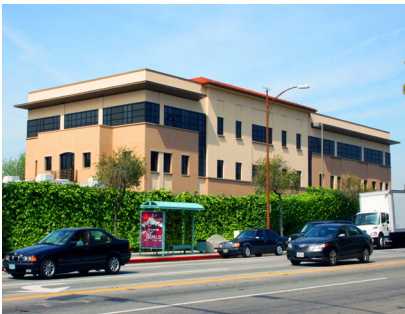
Warner Bros., Ranch Facilities (Building 2R) Burbank, CA
